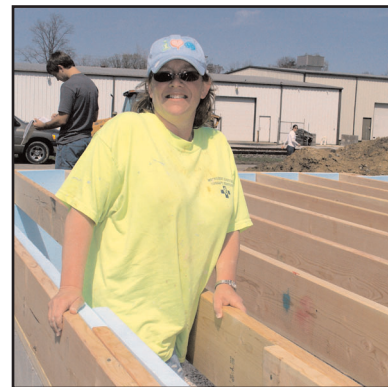
Chris Kinsey stands among the floor joists of her new home, sponsored with funds from the Melvin Dickhaut estate.
