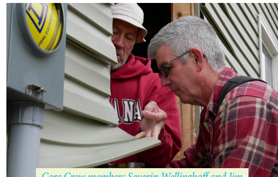
Core Crew members Severin Wellinghoff and Jim Havens install trim on Aysha's home
