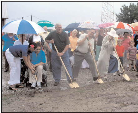
Partner family Lori Espenlaub, seated, helps to break ground on her new home in New Harmony. The home will be the first Habitat home built in that community. Jane Blaffer Owen, who donated the lot, is pictured at right. Mike Staubitz, house sponsor, is pictured to the left of her.
