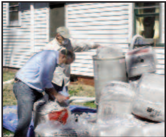
Most all the homes weatherized needed additional insulation in their attics. Pictured are two volunteers feeding insulation into the blower.
