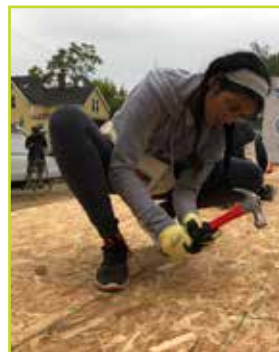
UE Student Volunteer, Vaishnavi Ravipati, helps build wall components.
